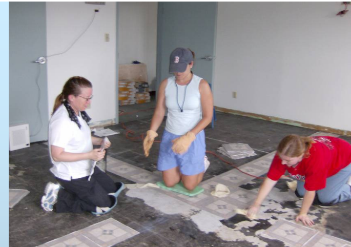
Katrina Work Team laying tiles in sister church
